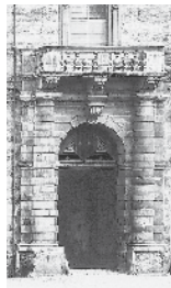
8. Forlì Detail of facade of Palazzo Paulucci
