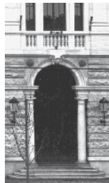
9. Rovigo Door of the Post Office building
