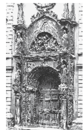
24. Ancona Gothic-Venetian door of the ex-Church of St. Augustine
