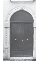
5. Campobasso Building in Via Sant'Antonio Abate
