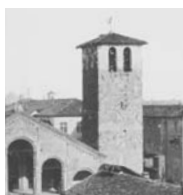
1. Milano Steeple, Basilica of Sant' Ambrogio
